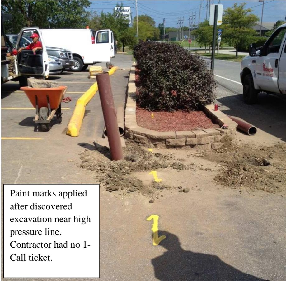
Paint marks applied after discovered excavation near high pressure line. Contractor had no 1-Call ticket.
