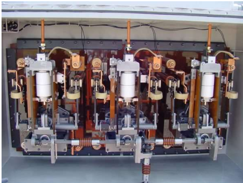
Figure 1. 3-phase Tap Changer. Adapted from "Understanding Load Tap Changers By Steve Skinner in Transformers, Circuit Breakers | August 23, 2017". Retrieved from http://www.artspphotoarchive.com/dancingindakota-112 . 2023
